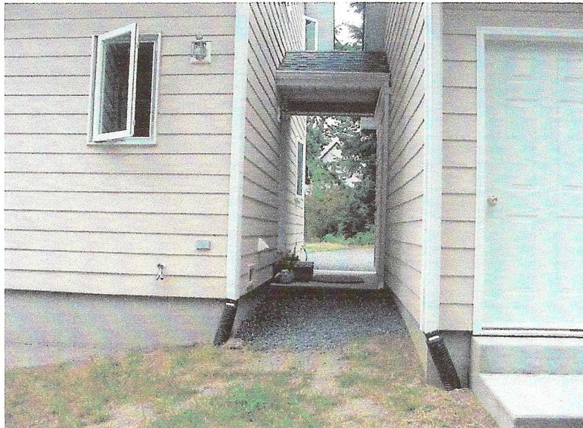
Gravel walkways and non-flammable building materials were used to advantage here.
